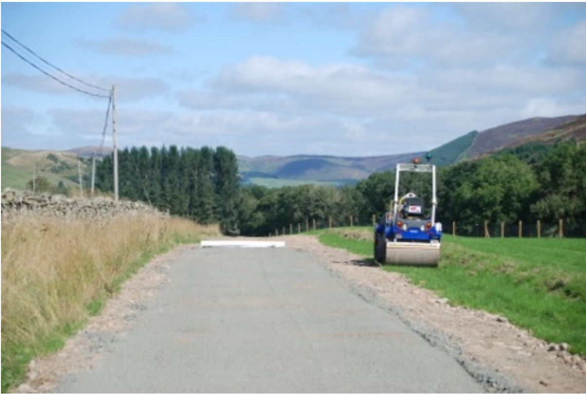
Photo 8 & 9. 26th August. New track being made by Water Board. Original pile of spoil used to level ground for track. Fibre membrane rolled out and then Grade 1 gravel laid.
