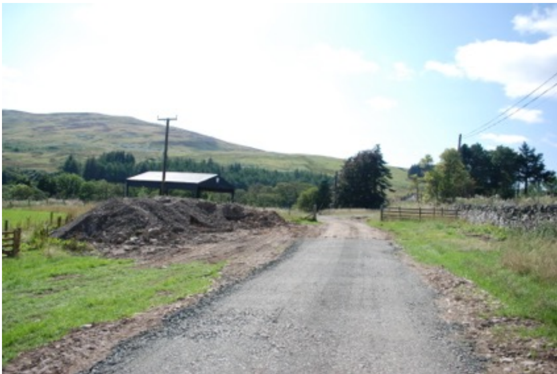
Photo 8 & 9. 26th August. New track being made by Water Board. Original pile of spoil used to level ground for track. Fibre membrane rolled out and then Grade 1 gravel laid.
