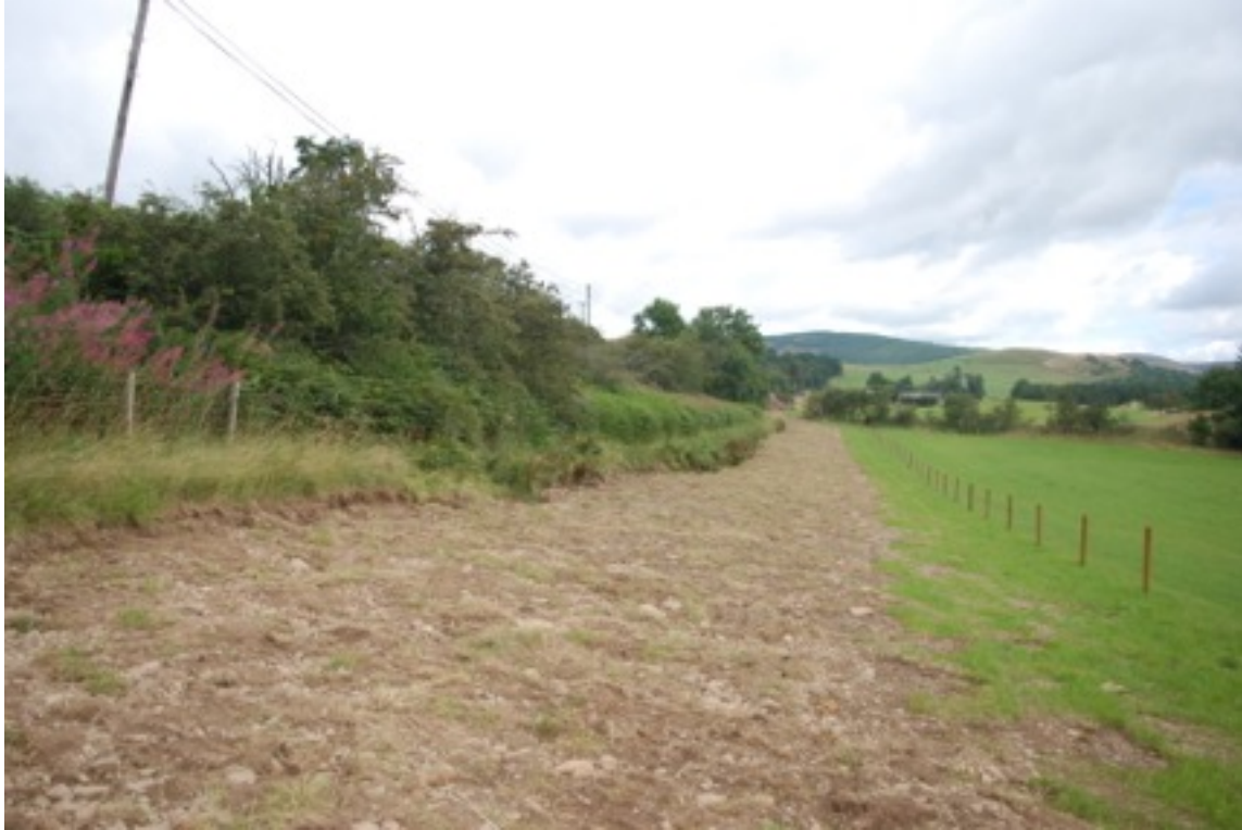
Photo 6. 16th August. East of old gate. Water Board reinstates earth and top soil after pipe has been laid.
